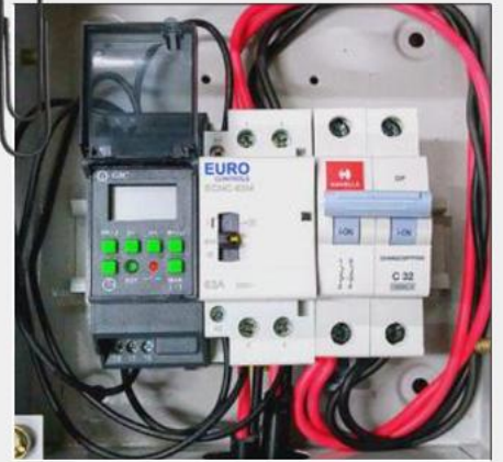
ONE STREET LIGHT FEEDER OF MC DALHOUSIE AUTOMATED BY FINAL YEAR STUDENTS ON SDM DALHOUSIE DIRECTIONS.
